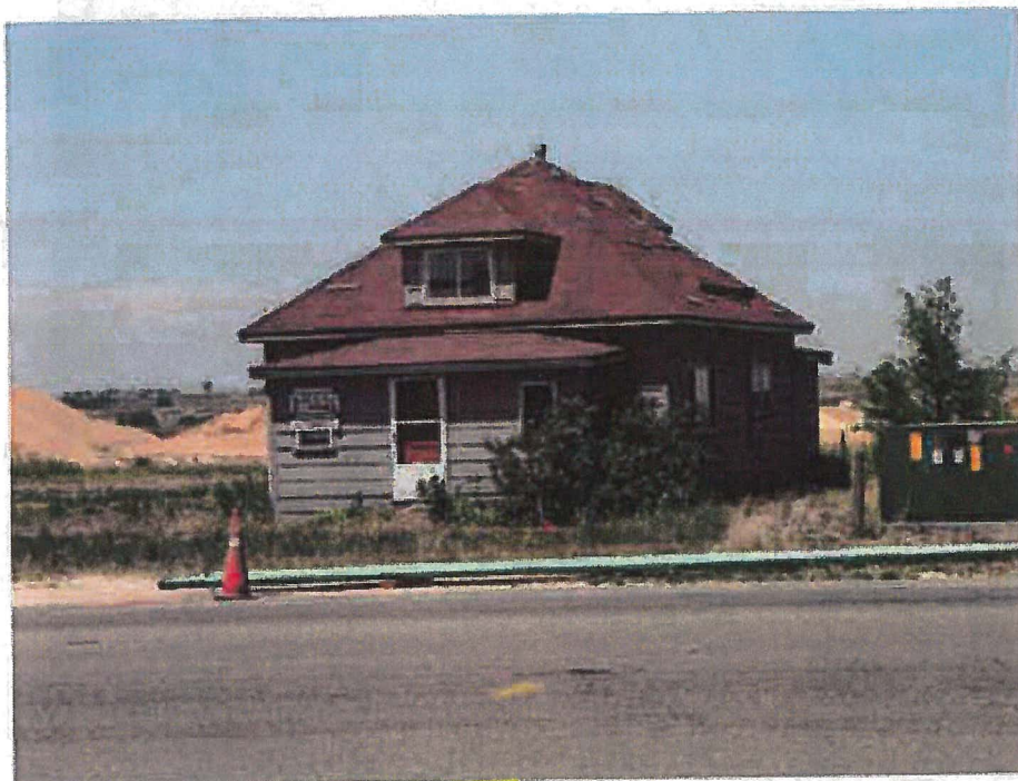
This vacant structure has deteriorated finishes
