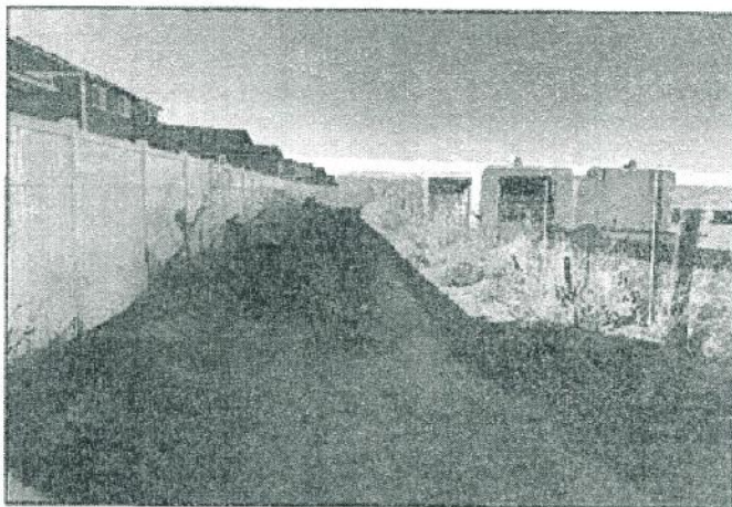
Photo 5 – low area at NW corner of Hopp property. Fill and excavation at west end prevents water from draining.
