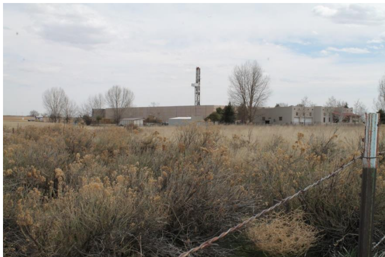
Figure 2-2 View southeast toward drilling site
