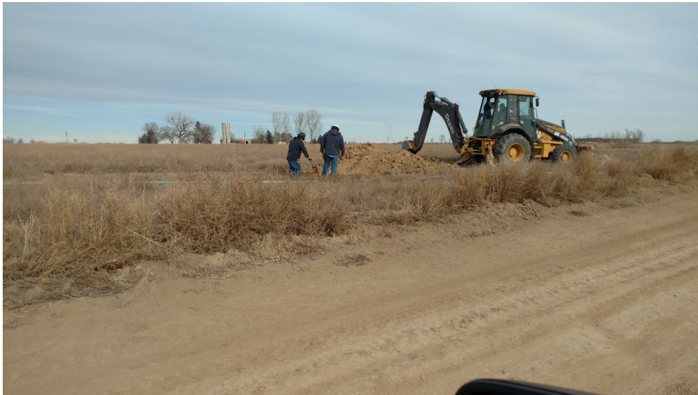
Figure 3 - Hamlin 4-36A Flowline Removal (January 9, 2019)
