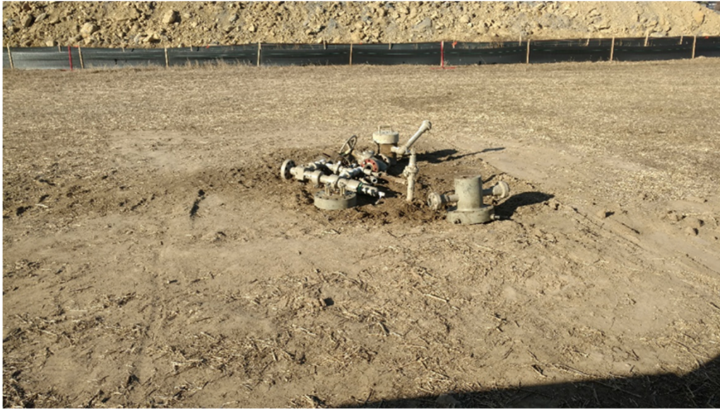
Figure 2- Hamlin 4-36A Well P&A Completed (December 19, 2018)
