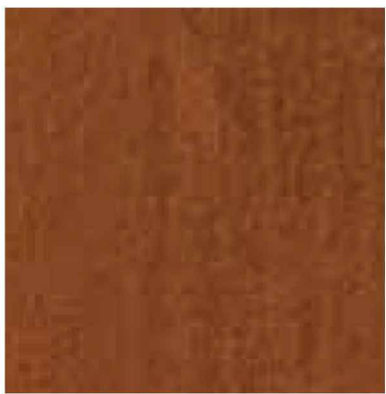
P1 - Rusted Metal
