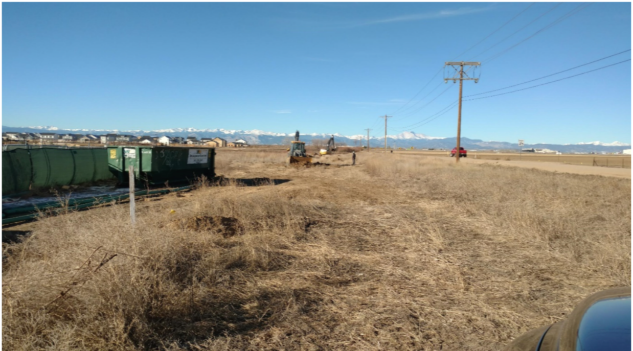
Figure 4- 4" Steel Natural Gas Gathering Pipe Being Removed Along South Side of WCR 28 East of Eagle River Road Extending to the East Side of WCR 11 and Under WCR 11 to the North.
