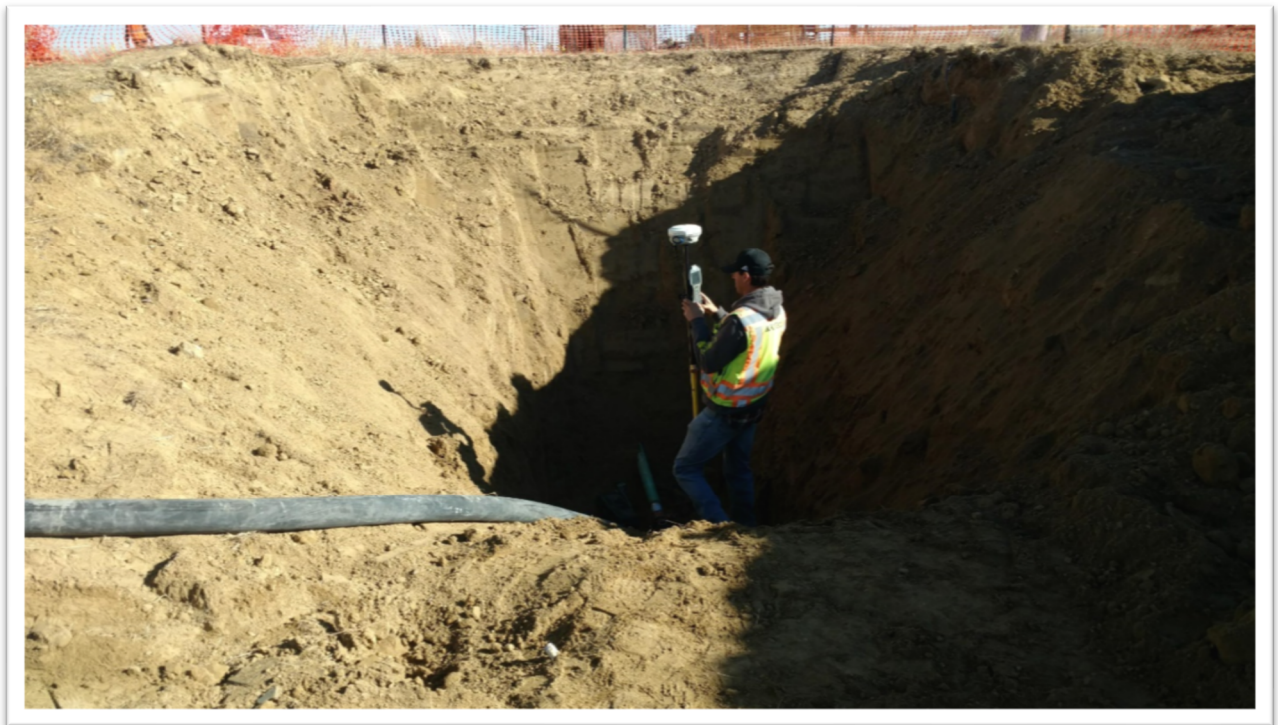
Figure 2 – Land Surveyor Collecting Exact Location of End of 4" Steel Natural Gas Gathering Pipe in Filing No. 1. The Black Hose Was Used for Flow-Filling.
