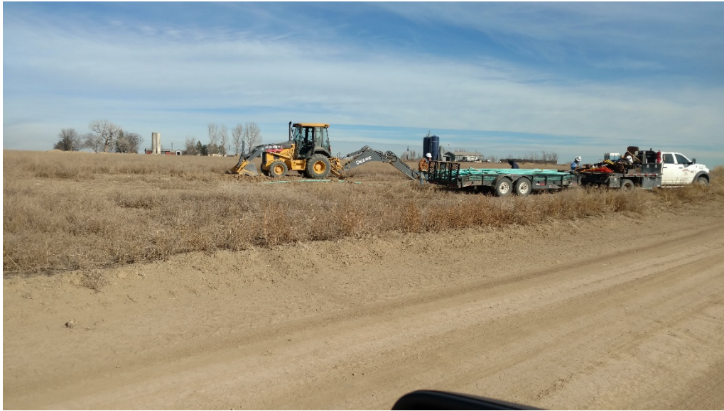
Figure 4 - Hamlin 4-36A Flowline Being Hauled Away (January 10, 2019)
