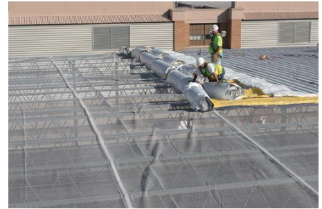
Sky-Web® Fall Protection and Insulation Support System protects workers from falls from the leading edge of the roof while also protecting workers below from dropped tools. It increases worker productivity while improving safety. After construction it serves as a virtually invisible insulation support system.
