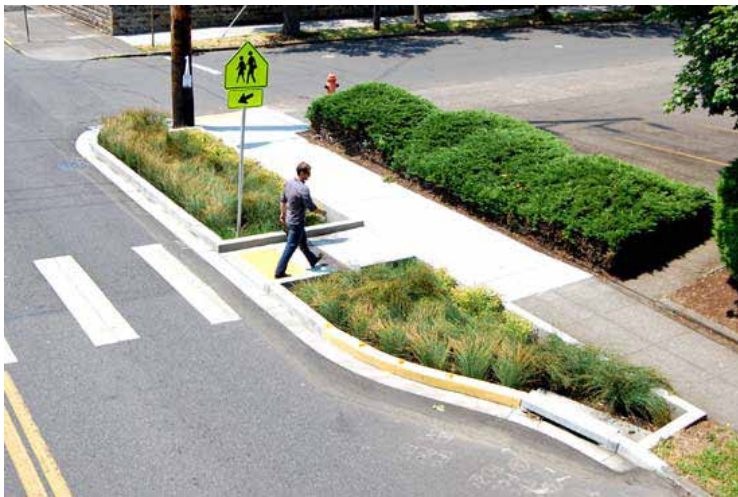
Bulbout and landscaping at pedestrian crossing.
