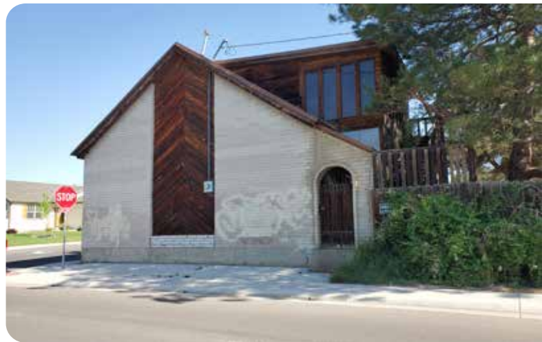
Historic Buildings, Former Screwball Inn
