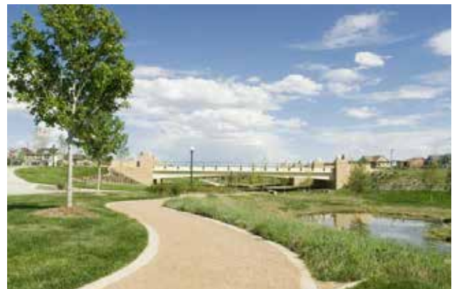
Off-street pedestrian trail.
