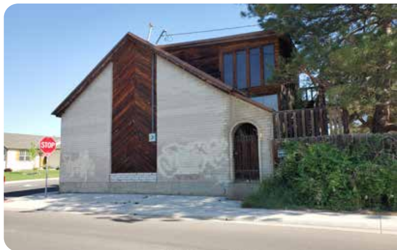
Historic Buildings, Former Screwball Inn
