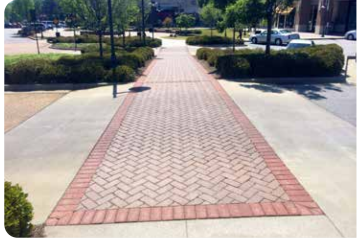
Paving materials used to help guide movement and differentiate between uses.
