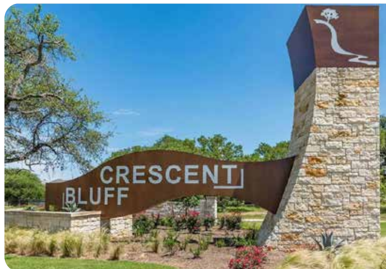
Steel and masonry materials and landscaping in gateway
