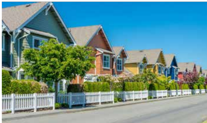
Buildings located to promote a continuous and uniform building frontage.
